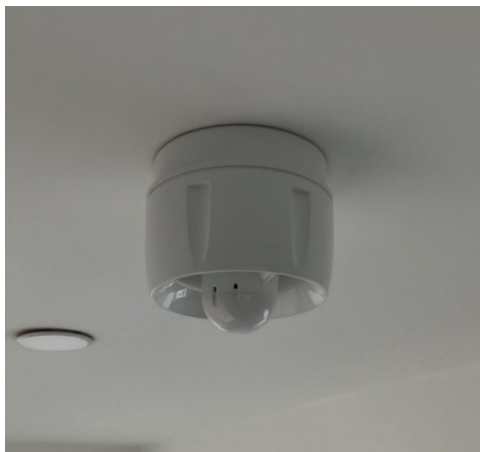
Fire evacuation alarm sounder located in ceilings
