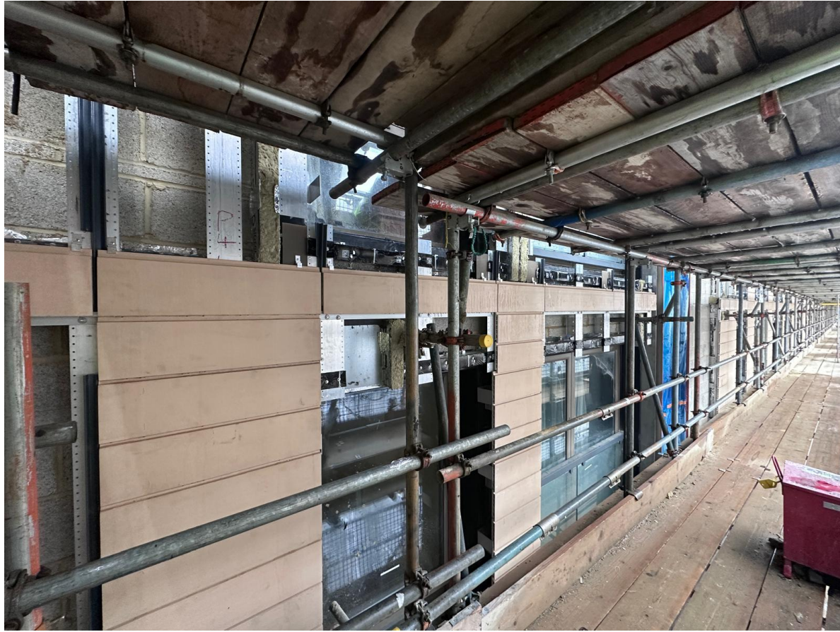
Phase 4 – Levels 2 to 8 – Terracotta Installation
