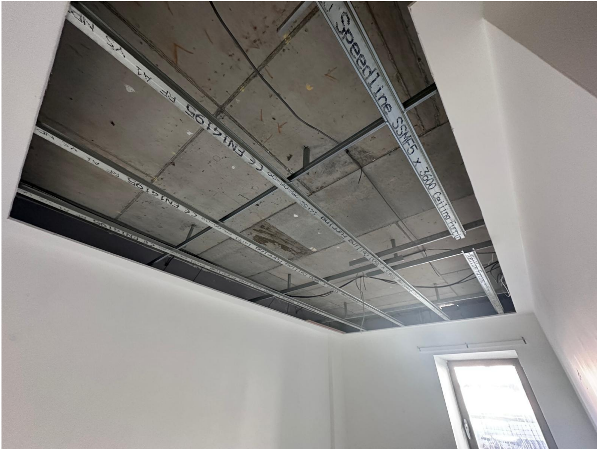
Old MVHR Ducting Removed
