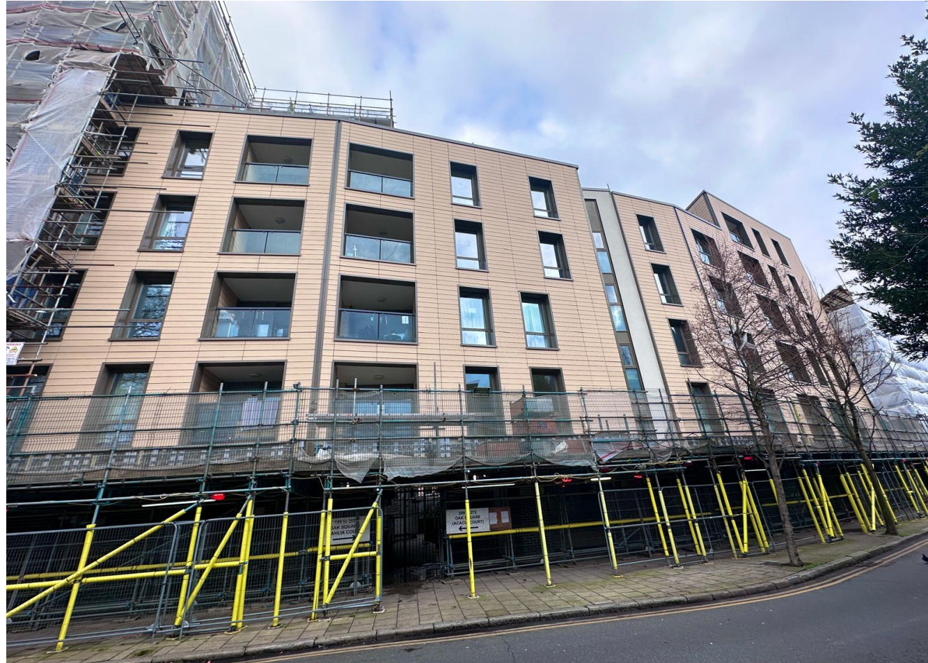
Phase 2 – Scaffold Struck to Gantry Level
