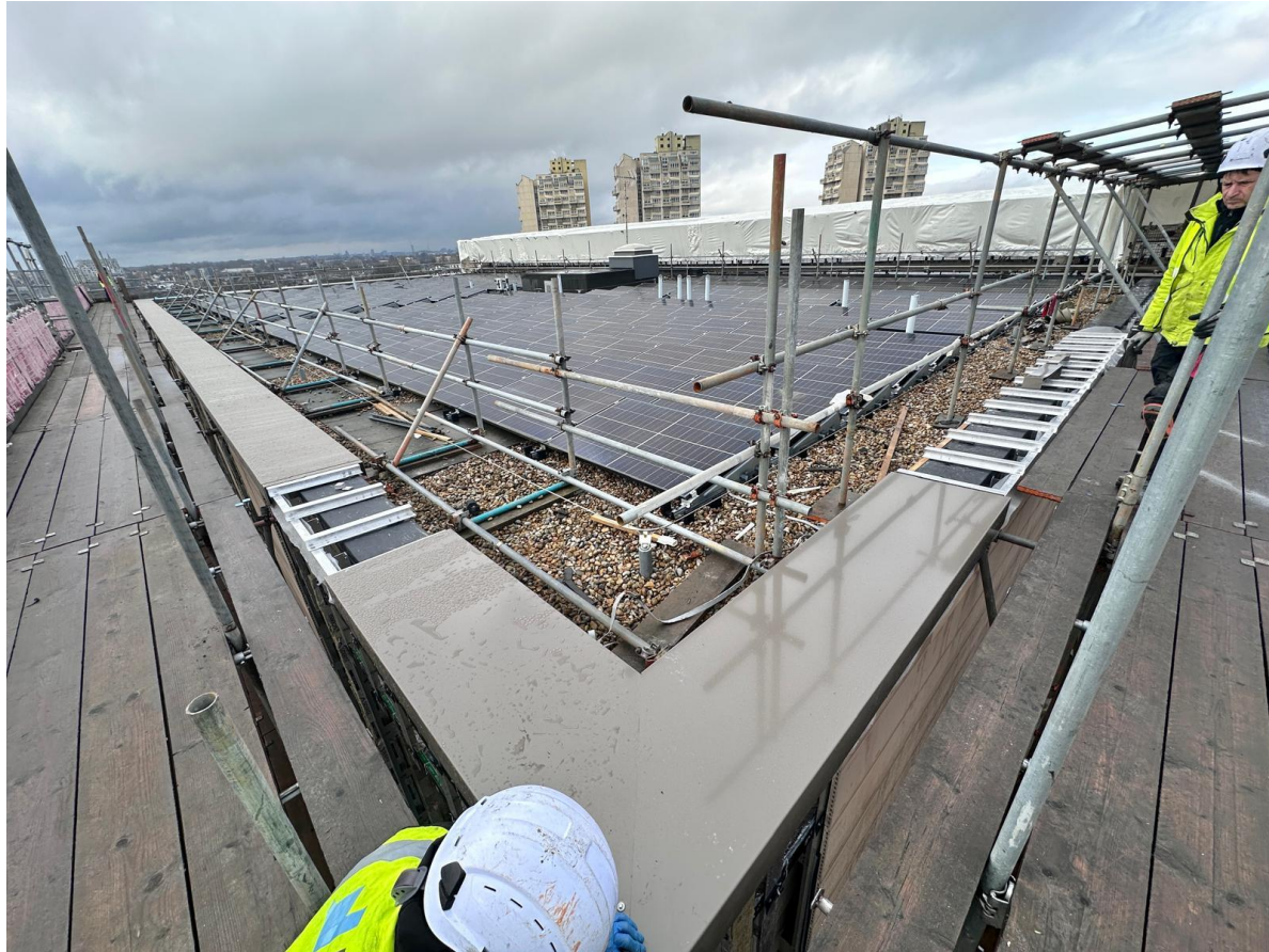
Phase 4 – Levels 1 to 8 – Roof Coping & Terracotta Installation
