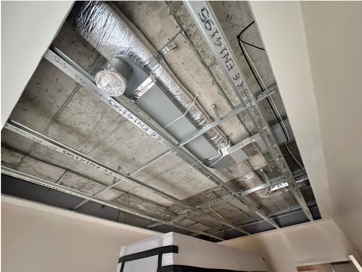
New Ducting Work Installed
