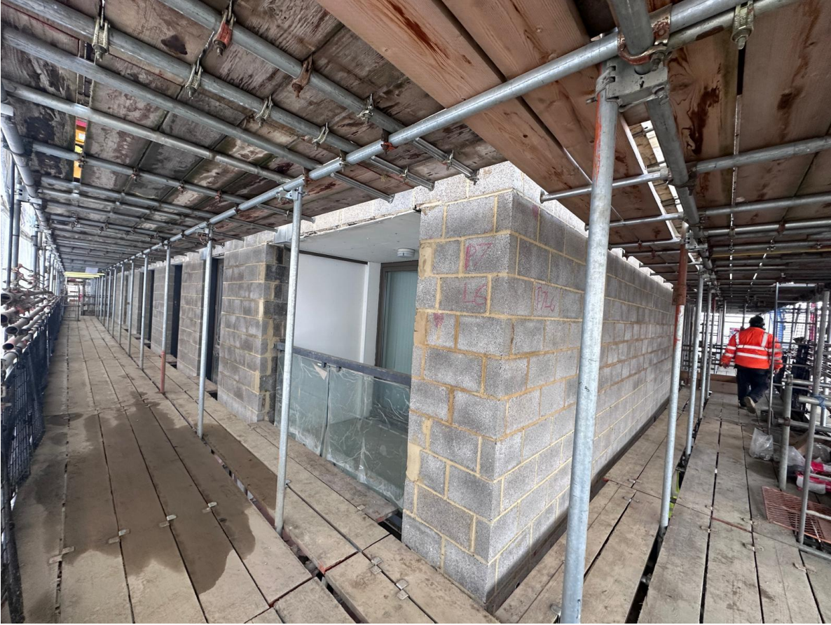
Phase 7 – New Outer Leaf Level 3 to 8
