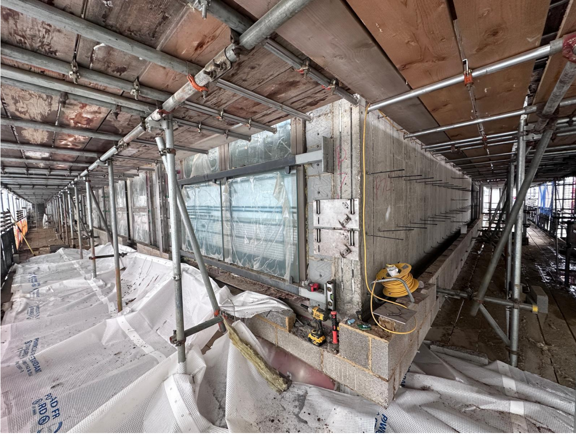
Phase 7 – New Outer Leaf Level 3 to 8
