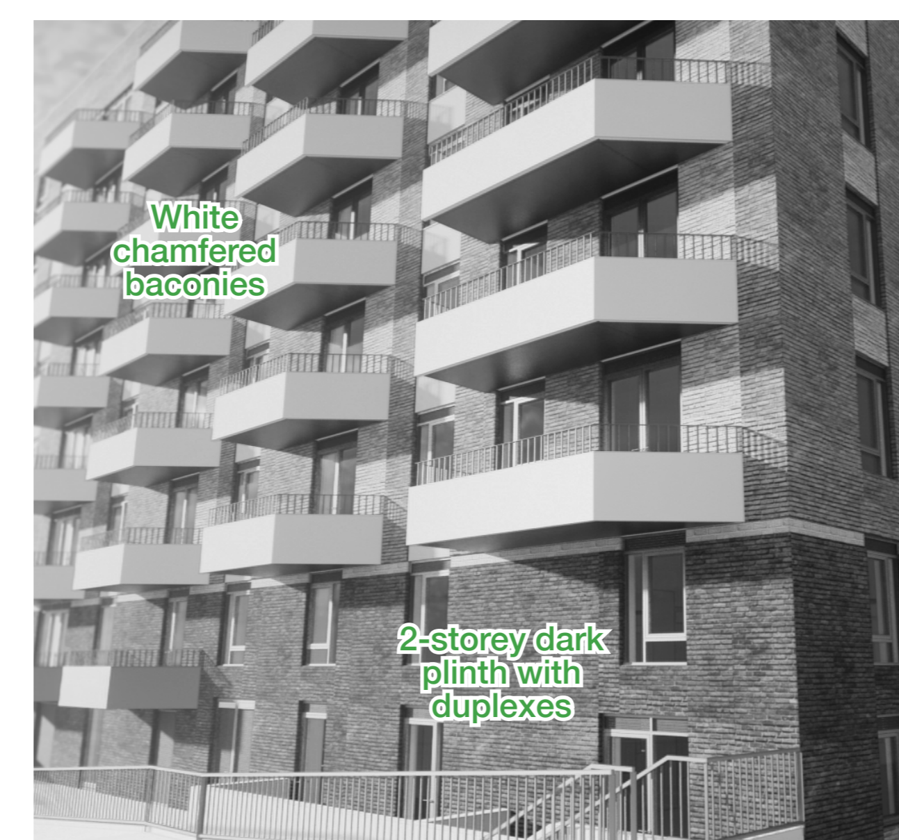
K2 Eastern balconies
