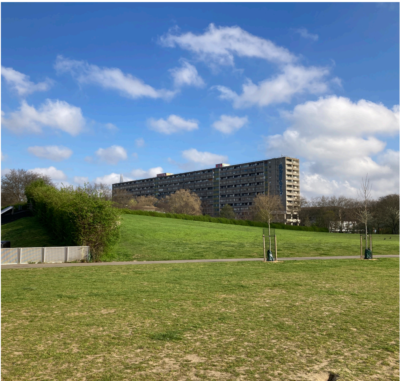
Figure 9: Aylesbury Estate, view from Burgess Park
