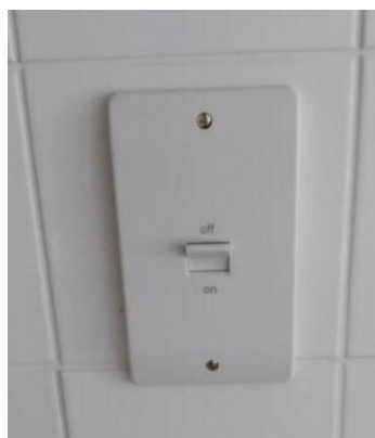
Cooker hood isolation switch – kitchen
