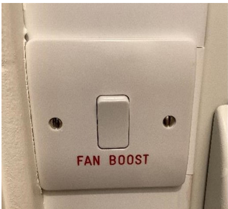
MVHR boost switch – utility cupboard
