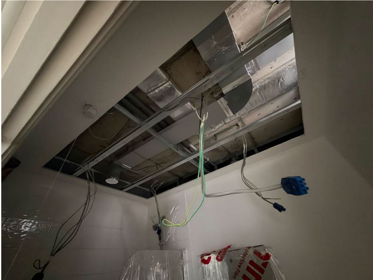
New MVHR Ducting Installed
