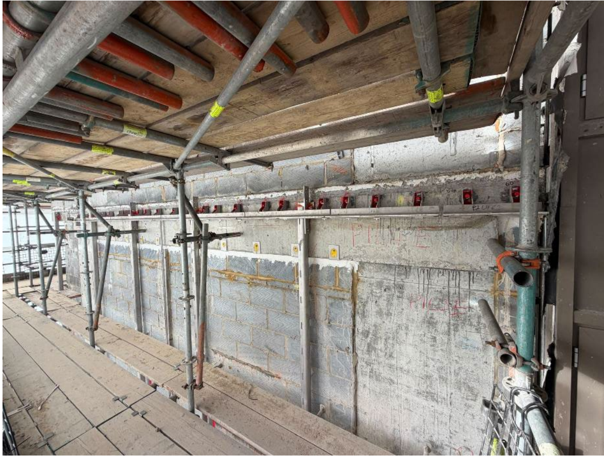
Phase 1 – Level 4 & 5 (East) – Masonry Support Installation in Progress
