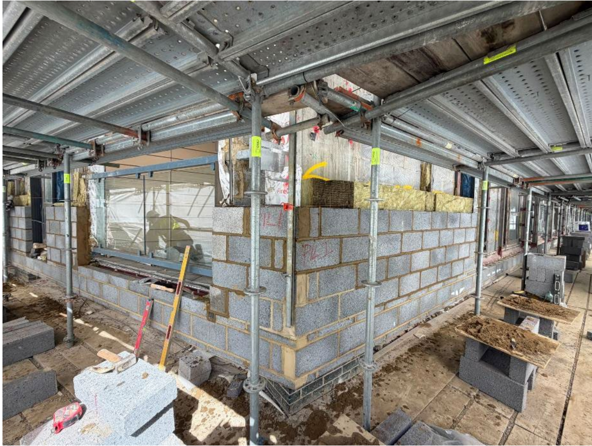
Phase 1 – Level 1 Outer Leaf in progress
