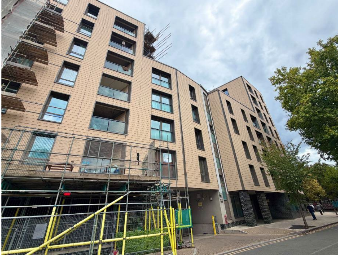
Phase 5W – Scaffold & Gantry fully struck.
