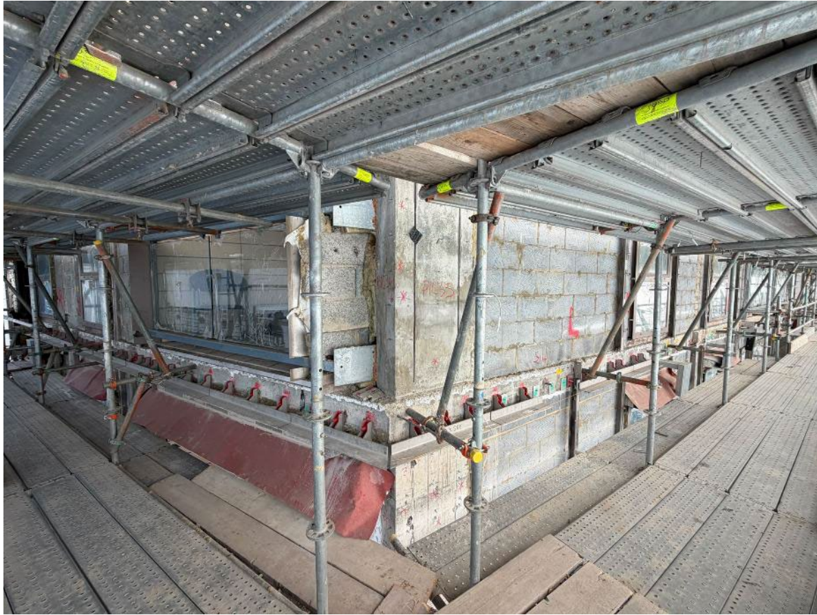
Phase 1 – Level 3 – Masonry Support Installation in Progress
