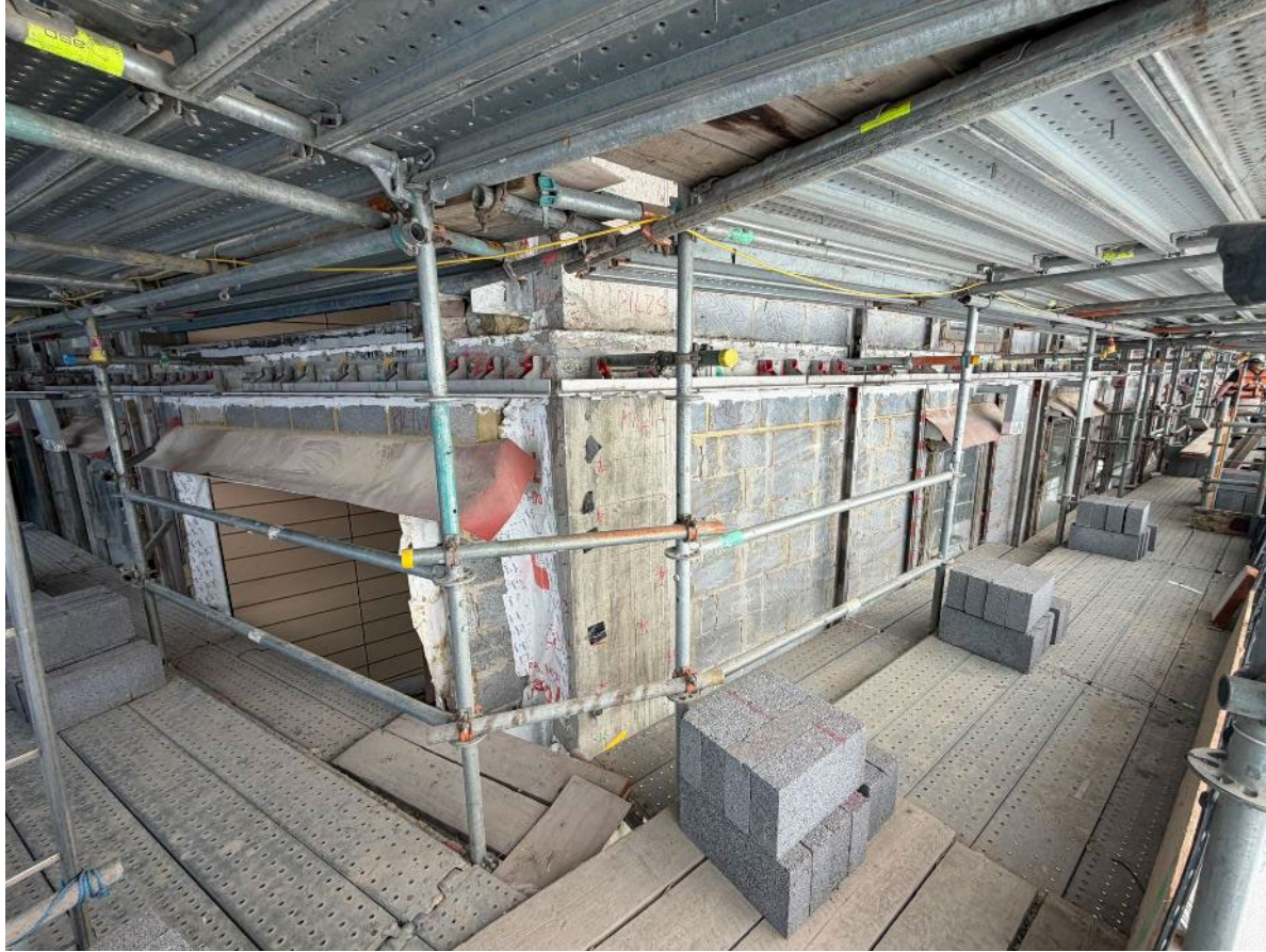
Phase 1 – Level 2 Masonry Support Installation completed and ready for Outer Leaf to commence.
