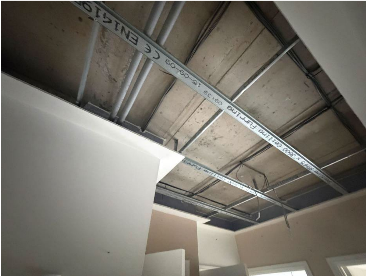
Ceiling Dropped and Old MVHR Ducts Removed
