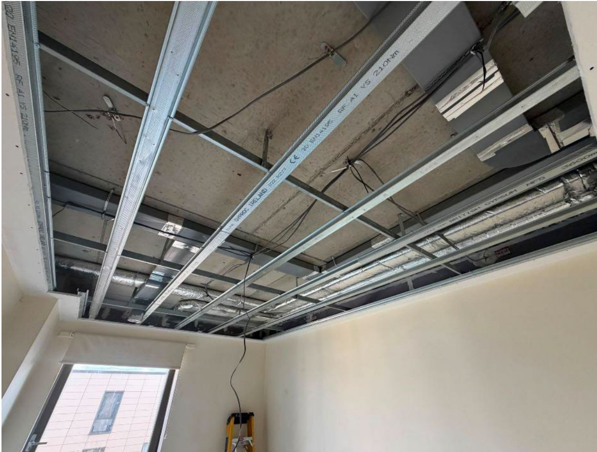
New MVHR Ducts Installed & Ceiling reinstatement progressing.
