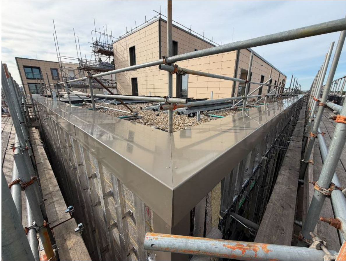
Phase 5N – PPC Copings Installed to Roof Levels
