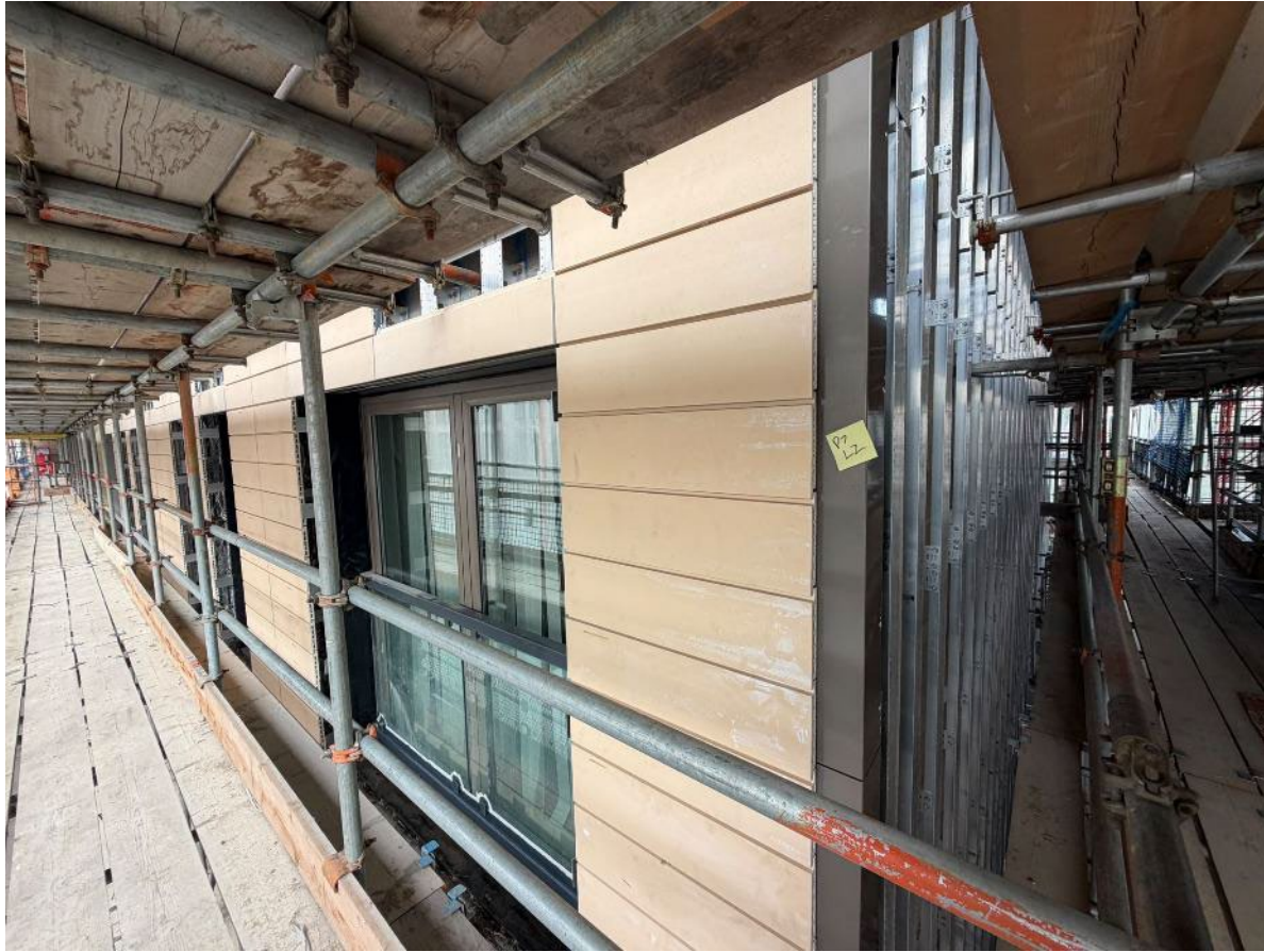
Phase 7 – Terracotta installation – Level 8 to Level 2
