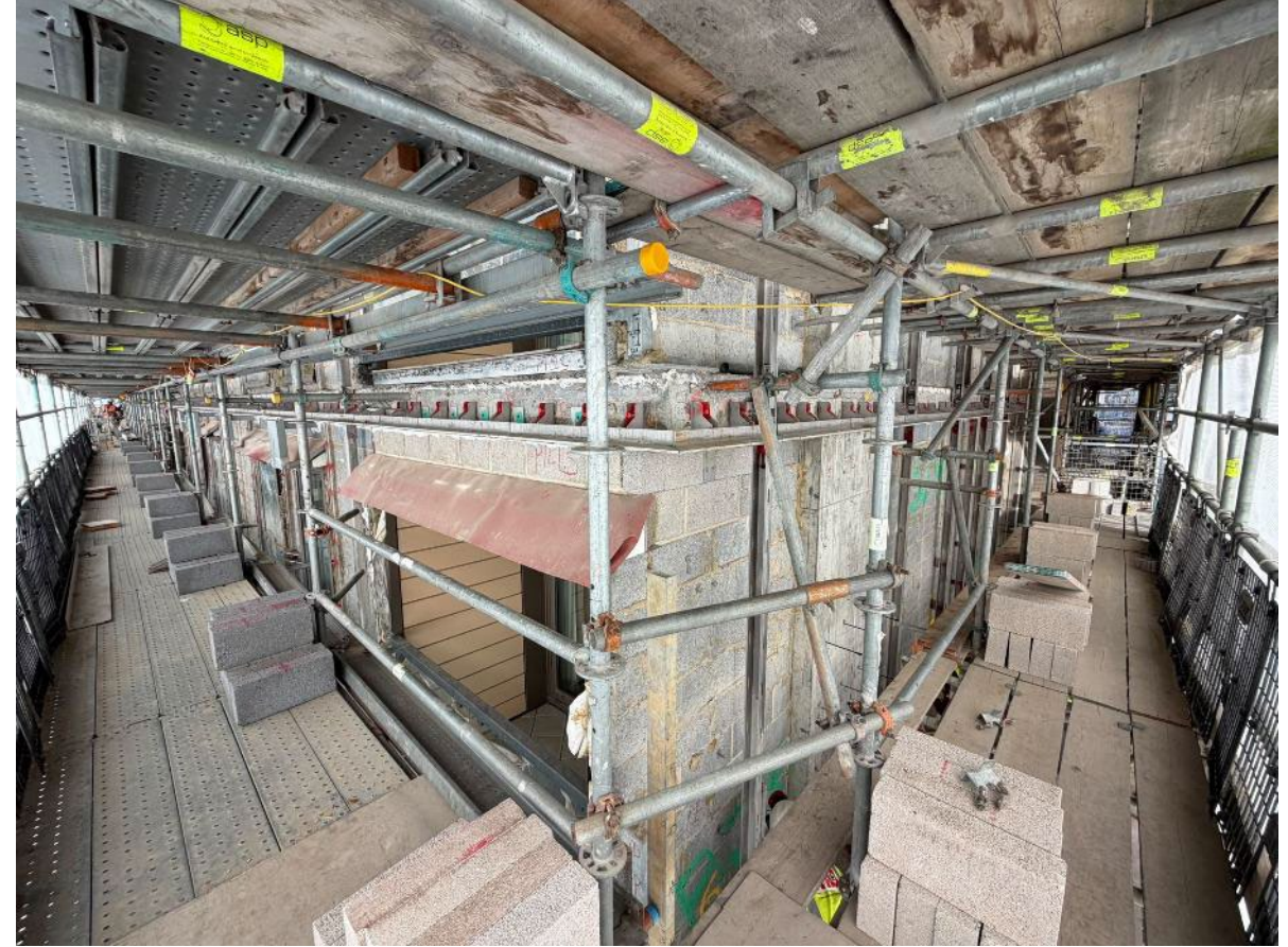
Phase 1 – Level 2 Masonry Support Installation completed and ready for Outer Leaf to commence.
