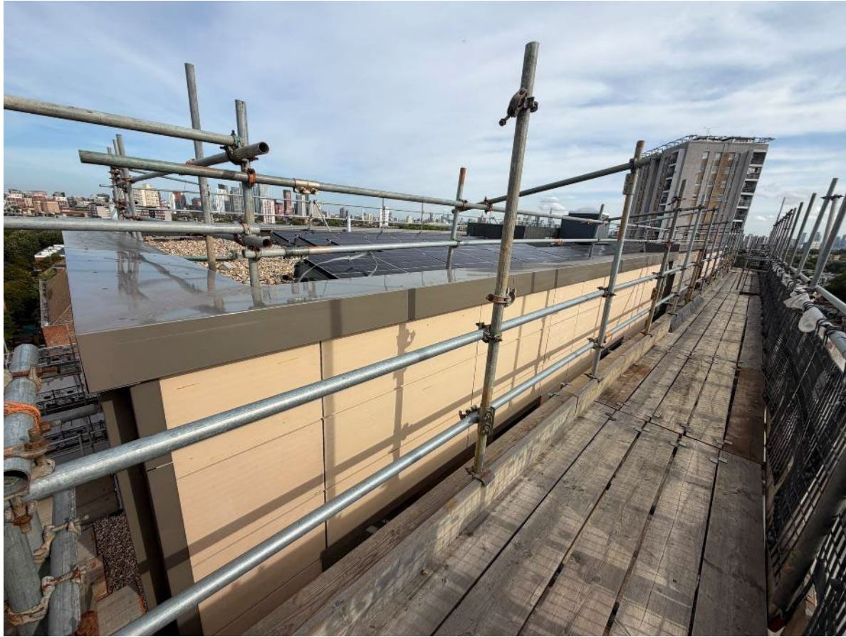
Phase 7 – PPC Copings Installed to Roof Levels
