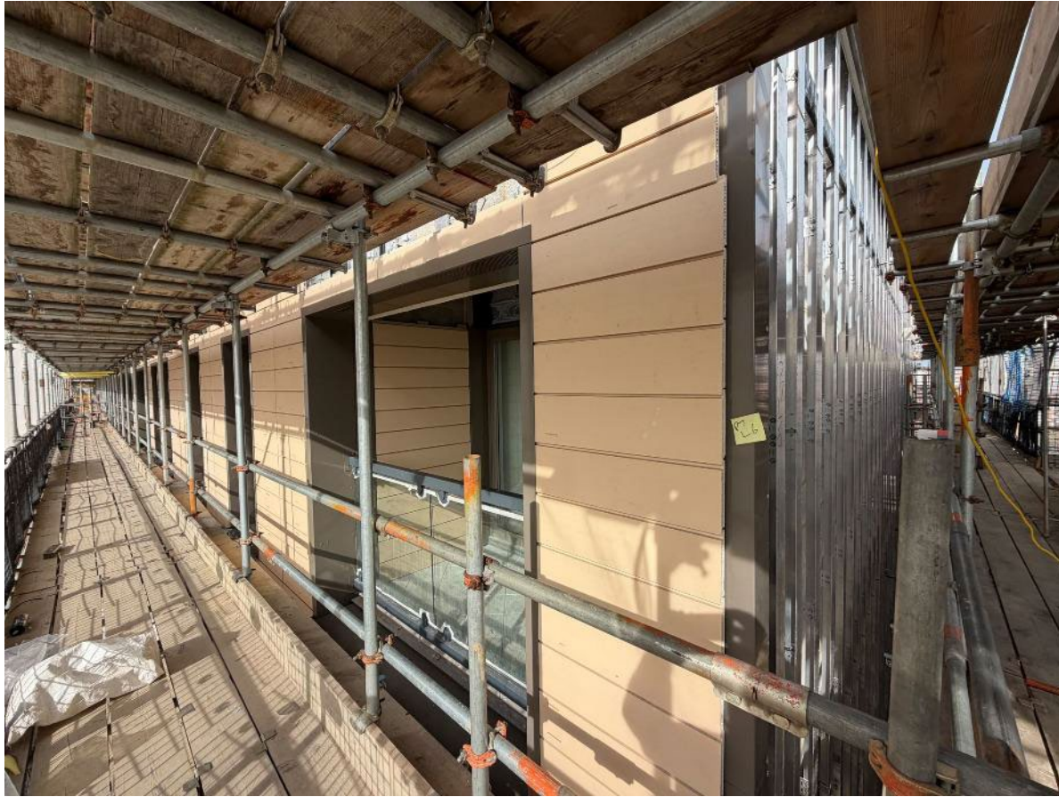
Phase 7 – Terracotta installation – Level 8 to Level 2
