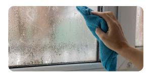
Condensation occurs when warm, moist air touches a cooler surface such as tiles, windows or walls. This causes the moisture in the air to condense, leaving water on these surfaces.
